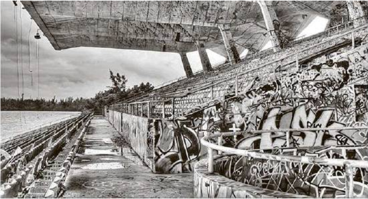
Miami Herald file A view of the graffiti-covered grandstand at the historic but long-shuttered Miami Marine Stadium on Virginia Key.
